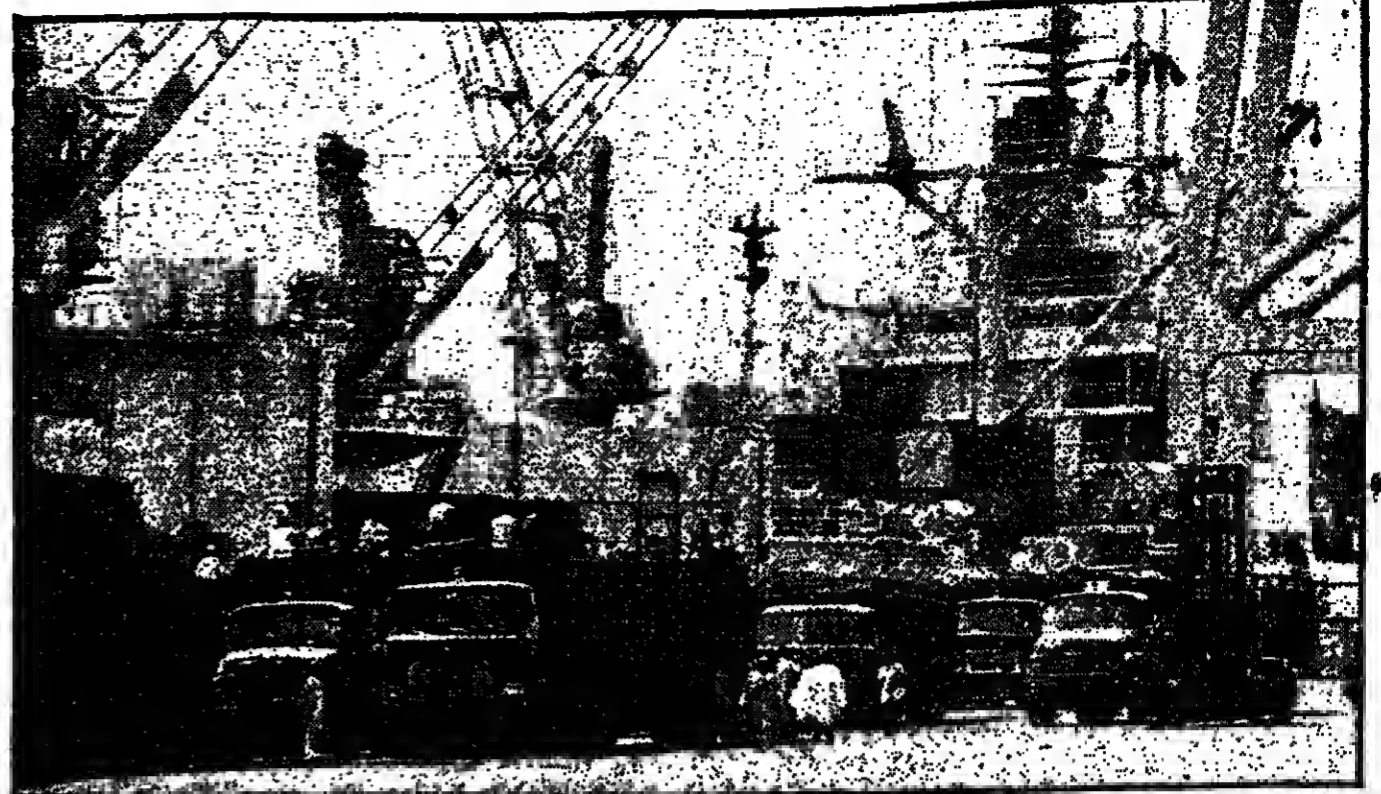
Cargo is unloaded at the third wharf extension at Apapa Keys, Lagos. Corruption in the ports has been greatly reduced but there is still a lot of pilferage and bureaucracy remains a big headache, claim port-users.
